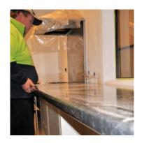
2. Check that the finished bench top has a gap of no more than 2 mm at any point to the wall. Fix it to the cabinets with screws, working from the underside of the cabinets' top rails. Be careful that the screws are long enough to provide a sound fixing into the bench top, but are short enough to avoid going right through.
