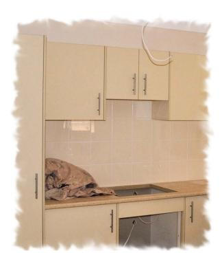
Apart from these clearance requirements, the height of the wall cabinets will also be influenced by the design and materials chosen for the splashback. For example, if the splashback behind the stove is going to be 4 rows of 150 mm tiles (as shown in the photo above) and you want to avoid cutting the tiles, the height would need to be 600 plus a grout width of 2 mm on either side of each tile – making it a total of 610 mm.
