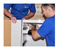
Fasten the floor units to the wall, using the appropriate fasteners for the material you're fixing to
