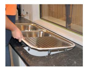
Put a bead of mould-resistant waterproof sealant around the top edge of the cut-out and place the sink on top. Then tighten up the clips. Wipe off any excess sealant that has oozed out with a damp cloth.
