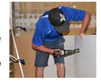
2. Place the cabinets one by one onto the plinth. In most cases, you'll find it easiest to begin with a corner unit and work progressively along the wall.
