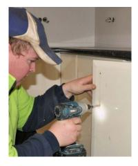
Mark the centre points for the screw holes by measuring down from the top of the door (or up from the bottom) and then in from the side.
