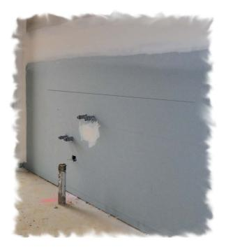
Once the height has been established, you should subtract the thickness of the bench top and then draw a horizontal line around the room to mark where the tops of the cabinets will finish. This forms the 'zero point', or reference line for the installation. For more details on the process of checking floor levels and deciding on the height of this line, go back to the unit: *Checking fit of cabinets*.
