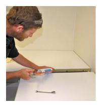
Never use glue to fasten the bench top to the cabinets. Glue doesn't allow for any movement that might occur due to variations in humidity or changes in temperature. The result is that the glue joint may fail over time, or alternatively the stresses may cause damage to the materials.
