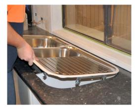
Put a bead of mould-resistant waterproof sealant around the top edge of the cut-out and place the sink on top. Then tighten up the clips. Wipe off any excess sealant that has oozed out with a damp cloth.
