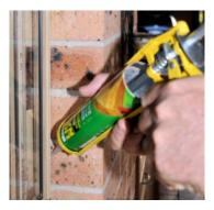
On the downside, polyurethane is toxic and emits fumes while it is being applied. It also needs to be cleaned up with a special solvent.
