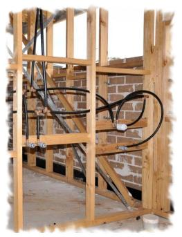
Most fixings for stud walls are designed to go into the studs themselves. However, for lighter loads, it is sometimes possible to use fasteners that fix to the internal wall lining in between the studs – that is, in the wall cavity.
