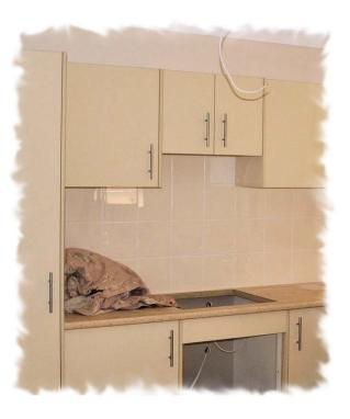
Apart from these clearance requirements, the height of the wall cabinets will also be influenced by the design and materials chosen for the splashback. For example, if the splashback behind the stove is going to be 4 rows of 150 mm tiles (as shown in the photo above) and you want to avoid cutting the tiles, the height would need to be 600 plus a grout width of 2 mm on either side of each tile – making it a total of 610 mm.
