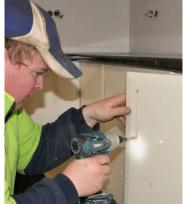
Mark the centre points for the screw holes by measuring down from the top of the door (or up from the bottom) and then in from the side.
