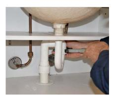
Plumbers look after all work involving water, gas, sewerage and wastewater. They need to work on the job before and after the cabinets are installed and tiling is done. Their first visit will be to run the pipes through the wall frames or floor, ready for the internal fit-out. Once the cabinets have been installed and tiling or other wall linings completed, they will come back to connect up the taps, sinks and other plumbing fixtures.
