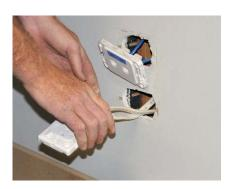
Electricians work with 'mains' electricity, often referred to as '240 volt power'. In some cases they also work with 'three phase' electricity, particularly in industrial buildings. Like the plumber, they need to come on-site before and after the cabinetry installation, firstly to run the wiring that will be needed and, when they return, to connect the appliances, power points and other electrical fixtures.
