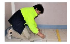
Not all kitchen projects use tiles, but just about every bathroom job does. This is because tiles are an excellent way of producing durable, waterproof and easy-to-clean walls and floors. Tilers generally work with ceramic or slate tiles, which are either glued in position or bedded in with cement-based mortar.
